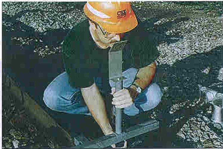
Figure 5-13: Looking through the peep hole to check the alignment
