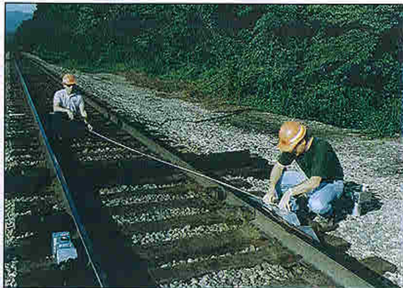
Figure 5-10: Maintainers using triangulation to ensure squaring of the scanners
